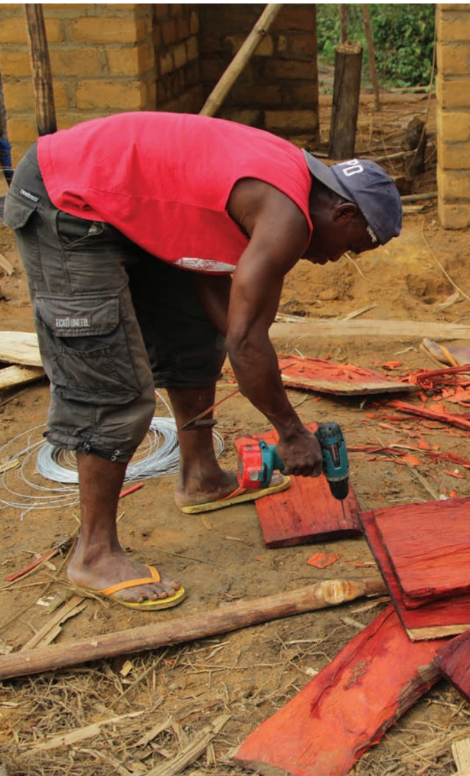
The roof shingles are made from a local hardwood, minimizing the cost of having to ship non-native materials into the remote landscape.
